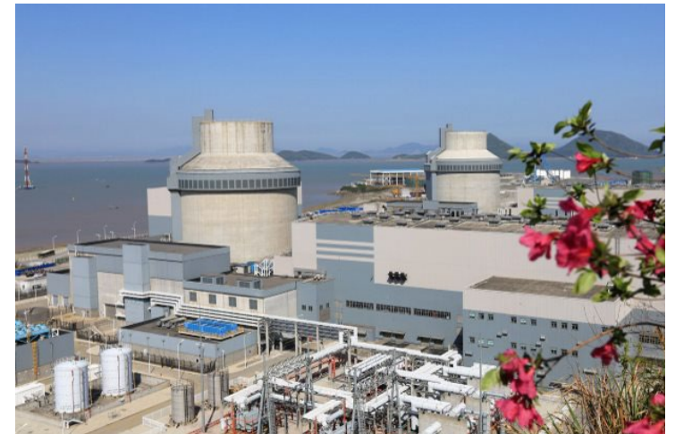
AP-1000 (Westinghouse) in Sanmen (CN), 1200 MW
