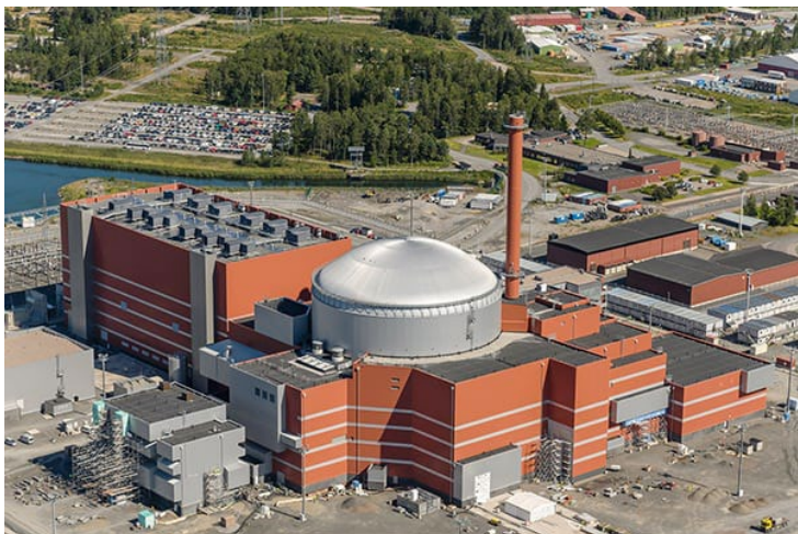
EPR (Framatome) in Olkiluoto (FI), 1600 MW
