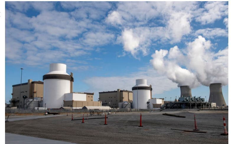
AP-1000 (Westinghouse) in Vogtle (USA), 2 x 1200 MW
