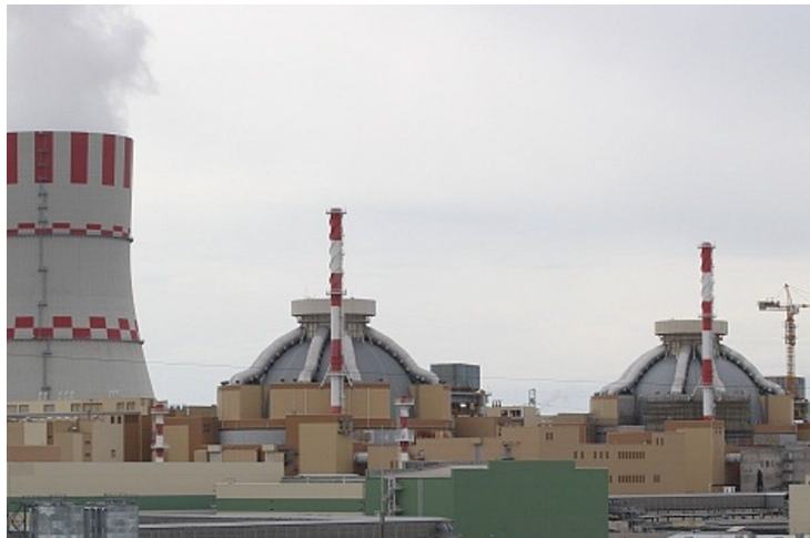
VVER-1200 (Rosatom) in Novovoronezh (RU), 1250 MW
