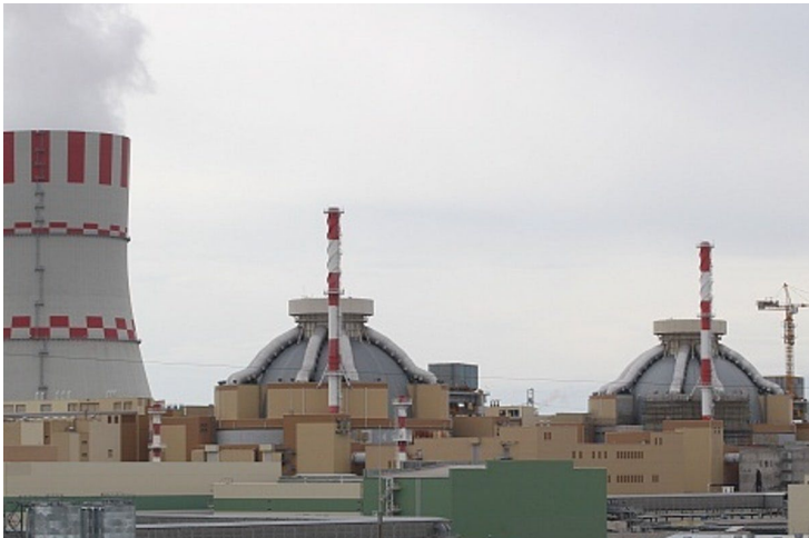
VVER-1200 (Rosatom) in Novovoronezh (RU), 1250 MW
