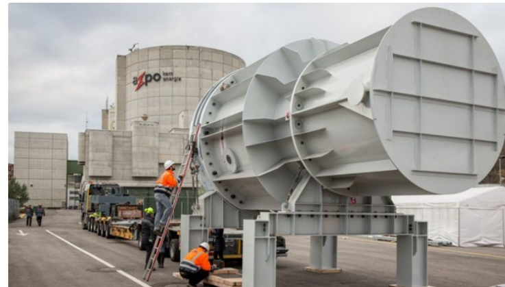
Exchange of Pressure Vessel Head in KKB
