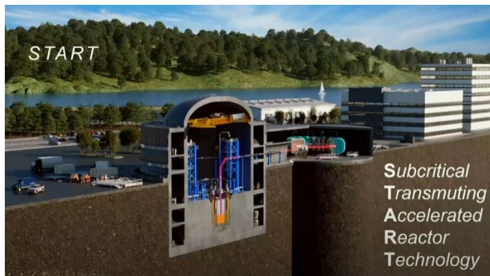
Transmutex START Reactor , a Swiss startup pioneering ADS/LFR technology for nuclear Waste transmutation
