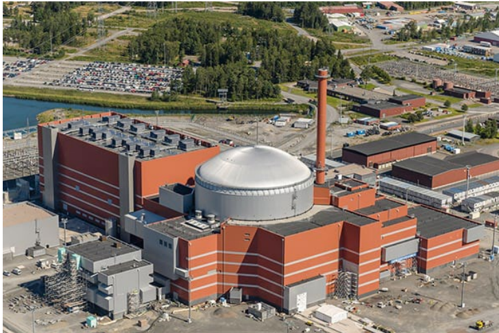
EPR (Framatome) in Olkiluoto (FI), 1600 MW
