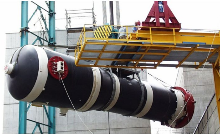
Exchange of Steam Generators in KKB
