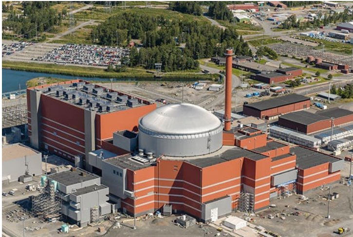
EPR (Framatome) in Olkiluoto (FI), 1600 MW
